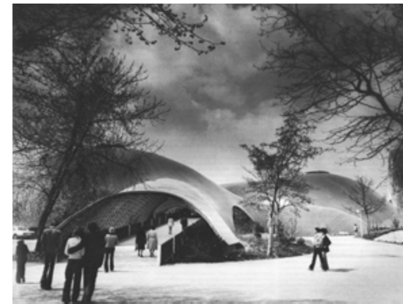
Figure 11: Multihalle mannheim. Flower exhibition Bundesgartenschau in 1975, Entrance area.
