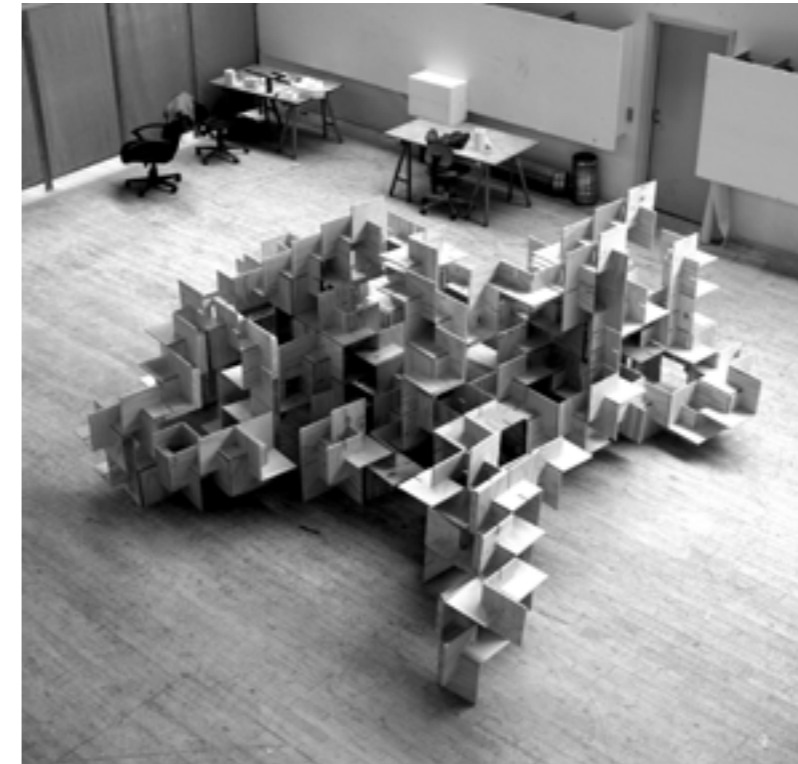
Figure 12: The realised SAGA structure. The structure gained a random expression. However, the rotational component type affected the tectonic expression substantially. The organic character, discovered via simulation, is also recognisable in the realised structure.
