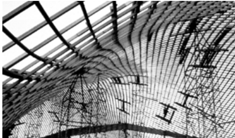
Figure 9: The process of erecting the structure was a complex task of gradually raising the supporting scaffolds and moving the lifting points, depending on the behaviour of the mesh.
