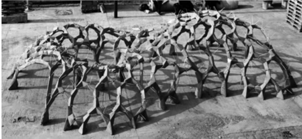
Figure 17: Case study three. Realised structure, Copenhagen. Photo: Ole E. Pedersen.
