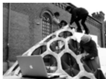
Figure 14: Figure 9: Case study two. Second assembly. The 3D model was used for referencing the components and the scaffold throughout the assembly process.
