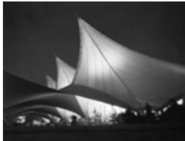
Figure 2: Top: Frei Otto. Soap film model of parallel wave tent. Above: Frei Otto and Peter Stromeyer's form-optimised tent construction for the Garden Exhibition in Hamburg, 1963. Photos: Institut für Leichte Flächentragwerke, University of Stuttgart.
