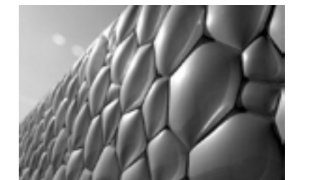
Figure 10: Right: The realised ETFE facade. Photo: Chris Bosse.
