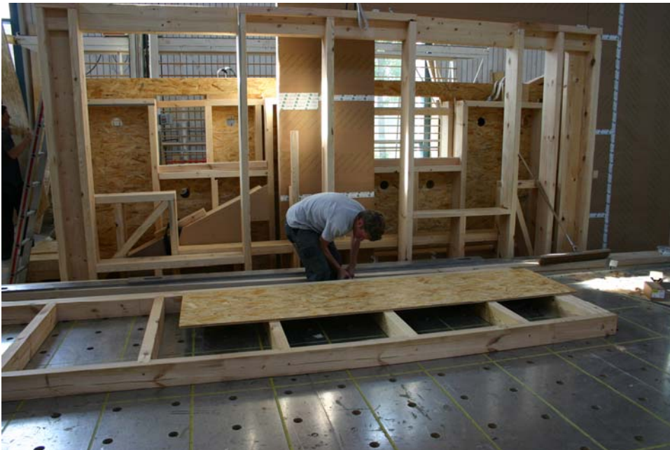
Figure 1 Wall assembly at the Berchtold Holzbau factory in Voralberg
