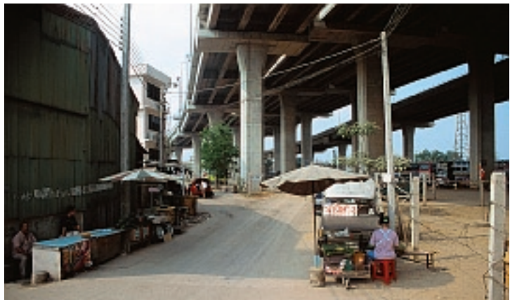
Residual space under the Inthra Expressway.
