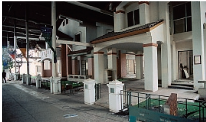
Inside the cracked "Expodome Home Center", Bangkok.
