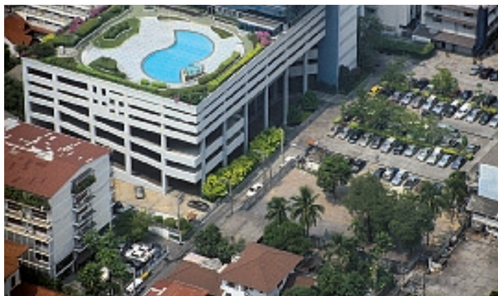
Typical pool-on-the-top parking structure, Bangkok.
