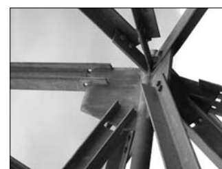
Fig 5B: Acoustic Barrier, ONL [Oosterhuis_Lénárd] 2004, File to Factory process of Mass-Customization generates 10.000 different nodes
